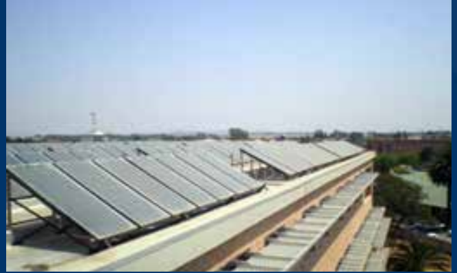
Industrial/ Commercial Bulk Water System
